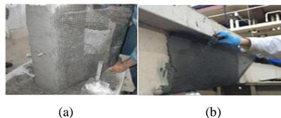
**Figure 5.** TRM as jacketing applications in a) columns and b) beams [69].
