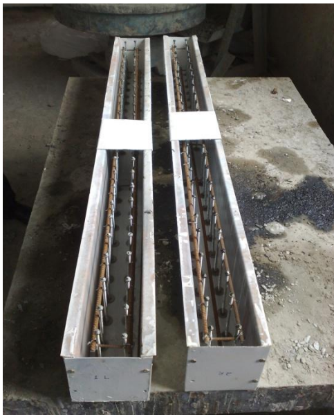
Fig .(3) Beam Reinforcement with Steel Mold
