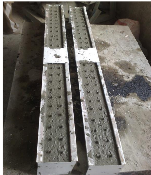
Fig .(4) Reinforced Concrete Beams after Casting in the Mold.
