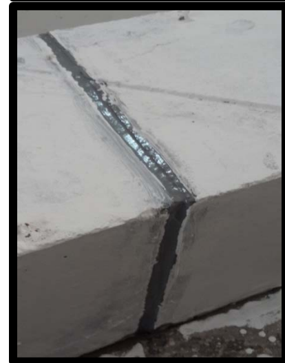
Figure 3. Epoxyed Joint for Beam SB6
