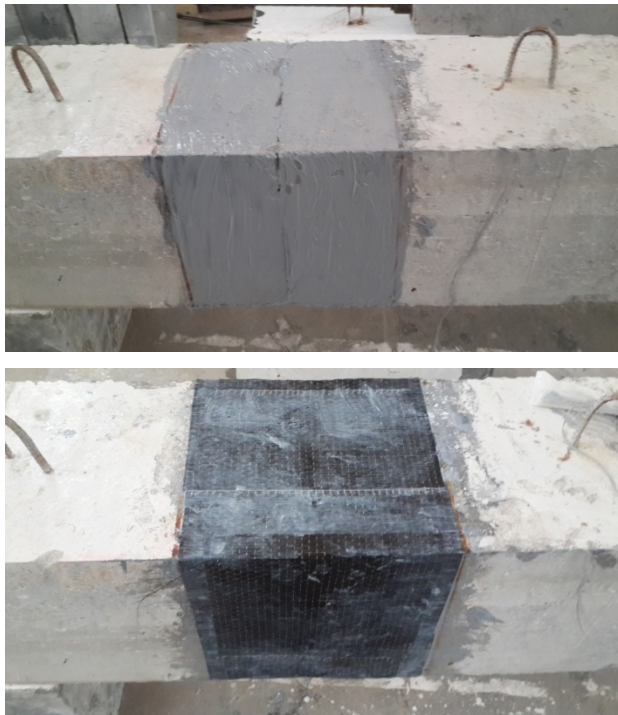
Figure 4. Dry Joint Strengthen by CFRP sheets
