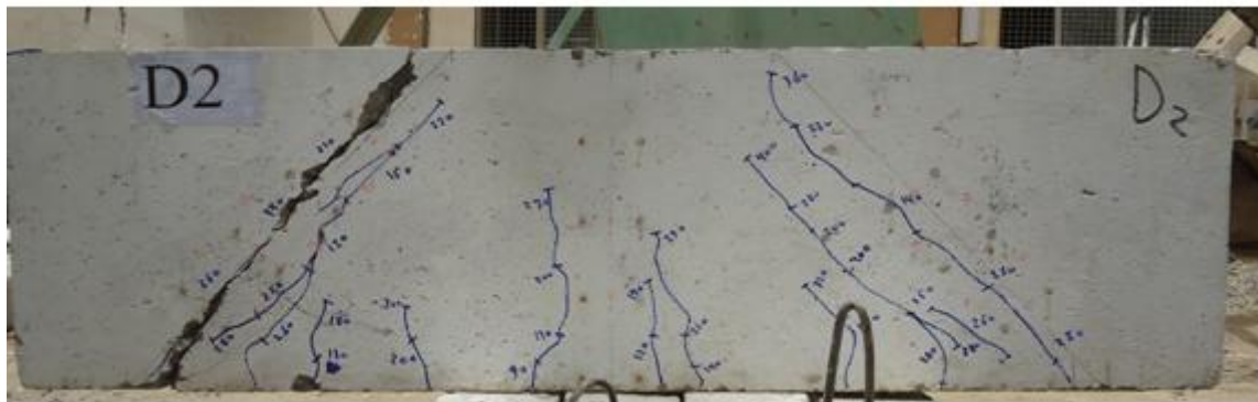
Fig .(9) Crack pattern for beam (D2)
