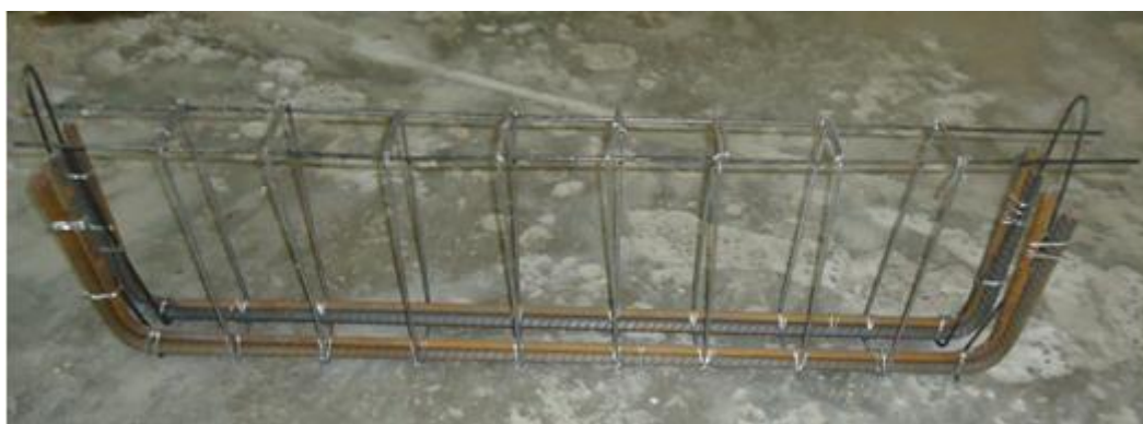
Fig .(1) Steel reinforcement cage used for tested beams
