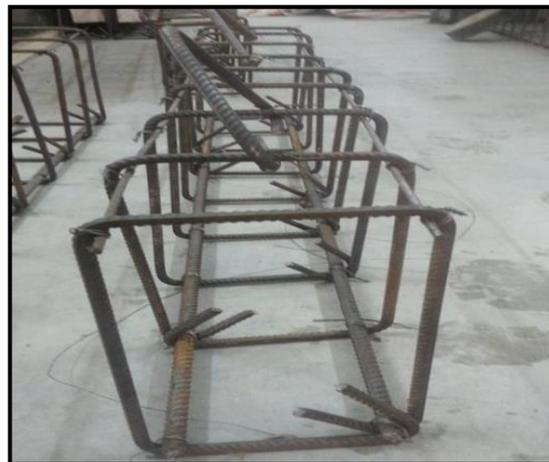
Figure 2. Details of Reinforcement
