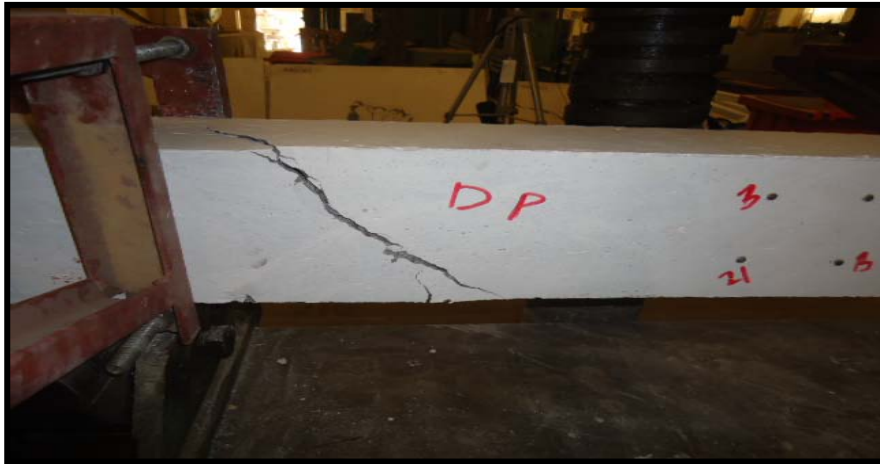
Figure (12), Crack Pattern and Failure Mode of Fibrous ( V_f=0.4\% ) SCC Beam (Dp)
