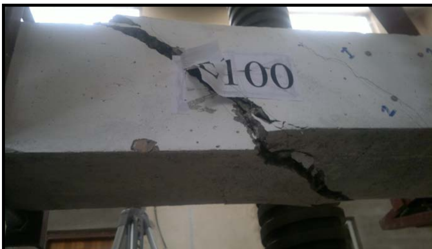
Figure (19), Crack Pattern and Failure Mode of Fibrous ( V_f = 0.8\% ) SCC Beam (E100)
