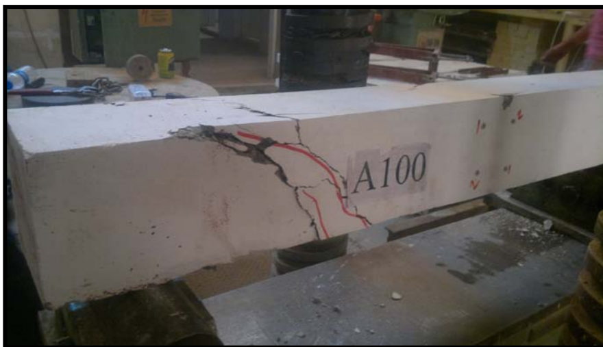
Figure (9), Crack Pattern and Failure Mode of Normal Strength SCC Beam (A100)
