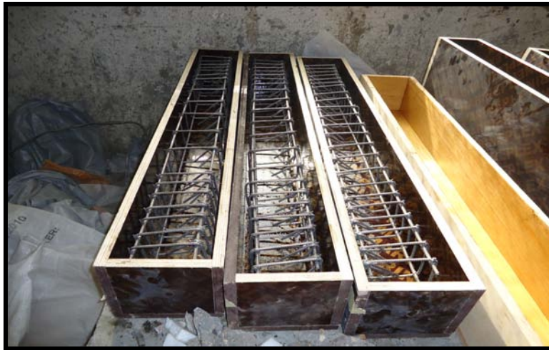
Figure(2) Steel Reinforcement and Wooden Mold
