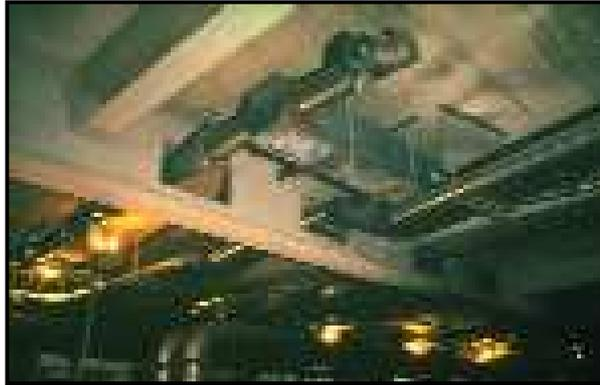
Figure1. Industrial Building (Openings through Stem of Beam)
