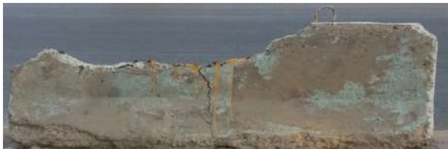
Plate(3) Concrete mass
