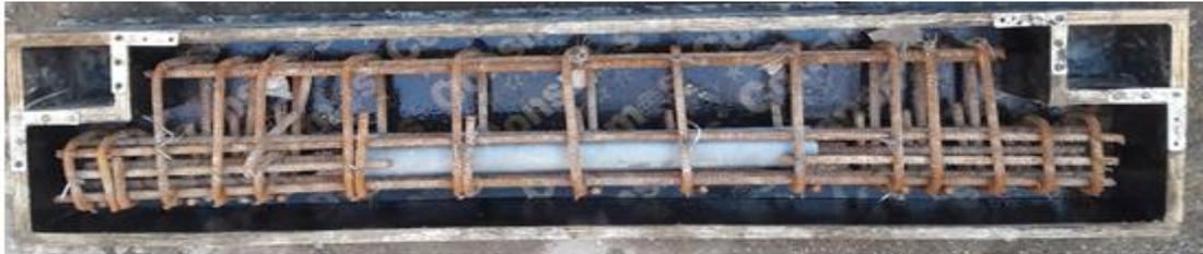
4. Mould & Reinforcement of R.C. Inverted Dapped Ends Girder, (DE4H)
