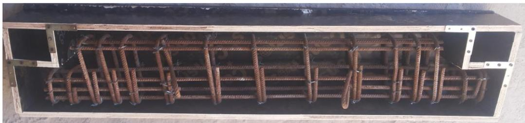
1. Mould & Reinforcement of R.C. Inverted Dapped Ends Girder, (DE1NH)
