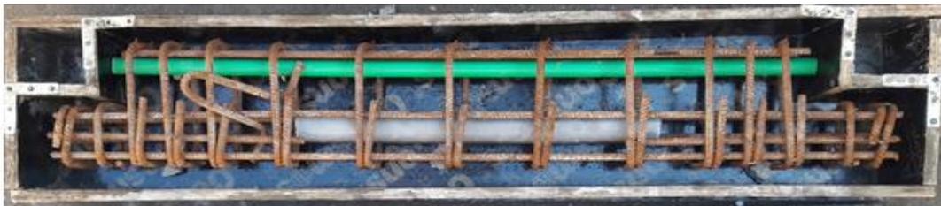
5. Mould & Reinforcement of R.C. Inverted Dapped Ends Girder, (DE5HP)
