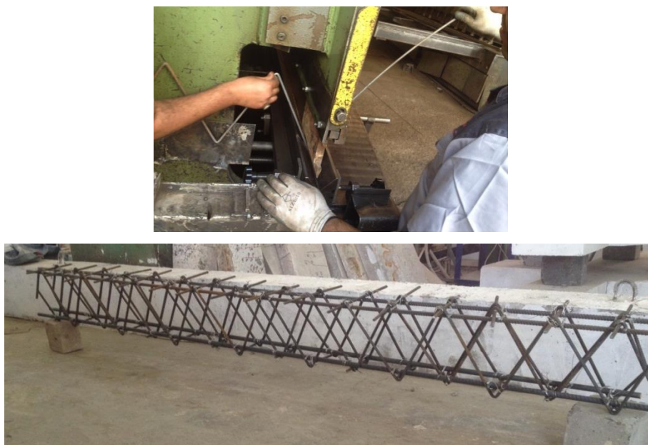
Figure 3. Lacing reinforcement fabrication.
