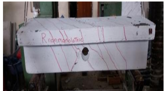
Plate 11. Specimen beam B8 – after test.
