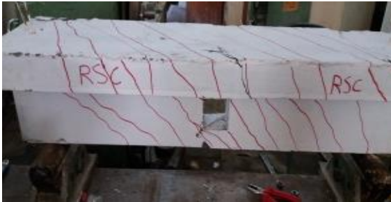
Plate 6. Specimen beam B3 – after test.
