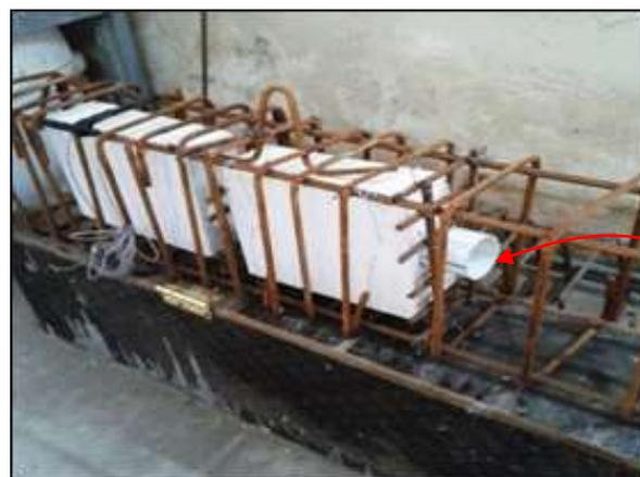
PVC Pipe between Polystyrene pieces to form Opening
