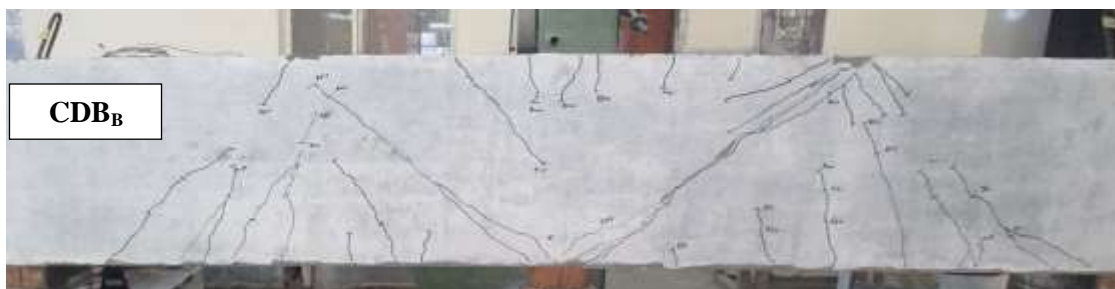
Figure 9. Crack pattern for beam CDB B after testing.
