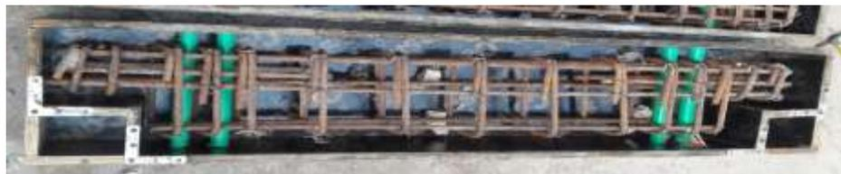
(E). Mold and Reinforcement of R.C. Beam Dapped Ends, (DE5)
