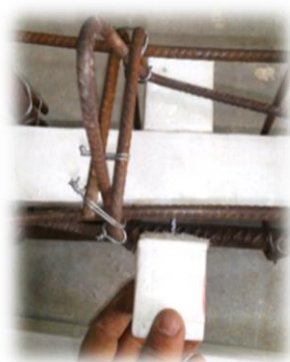
Fig (5): Preparing the Opening Mold (Top View).
