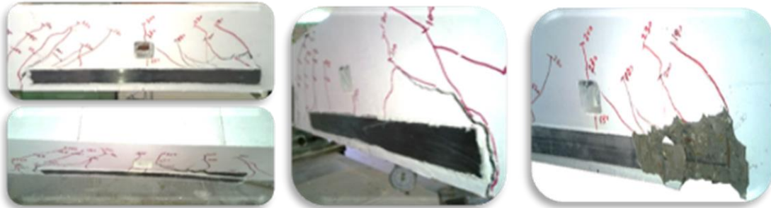
Fig.(19): Photographs of Concrete Ripping-Off by Flexural-CFRP Edges
