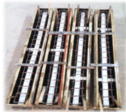
Fig (7): Molds Layout before Casting for BLTO Models
