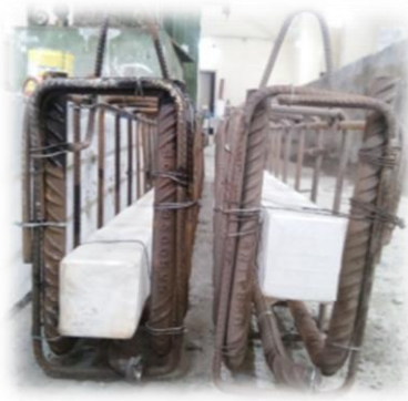
Fig (6): Hollow Core Location (Different Zone) in Reinforcing Steel Cages.
