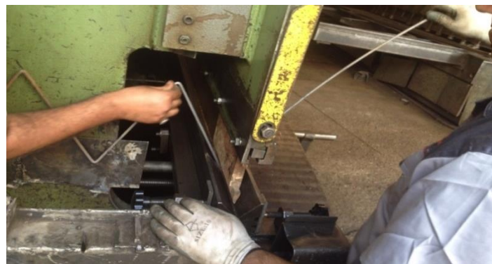
Fig. (3) Lacing reinforcement fabrication.
