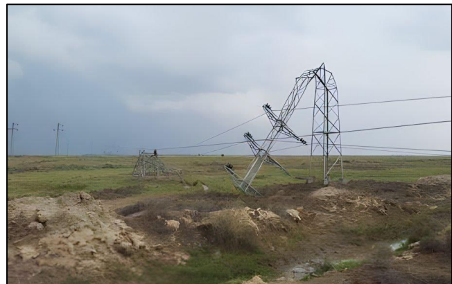
Figure 4. The case of the tower under study after a tornado.
