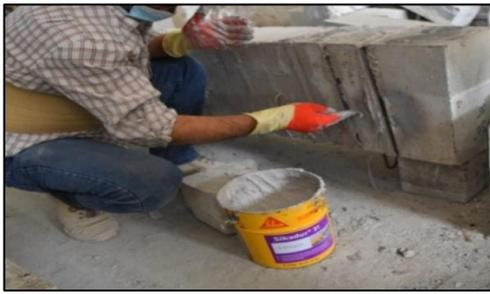
**Figure 4.** Strengthening by NSM Steel Bars
