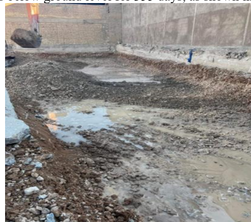
Figure 6. Preparing the location of the beams at a 2-meter underground level.
