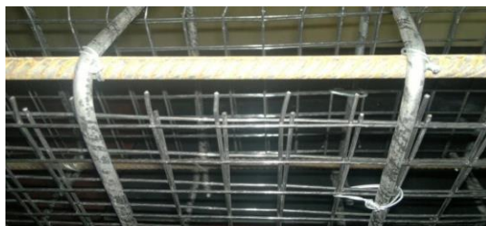
Figure 2. Steel meshes used in the work.
