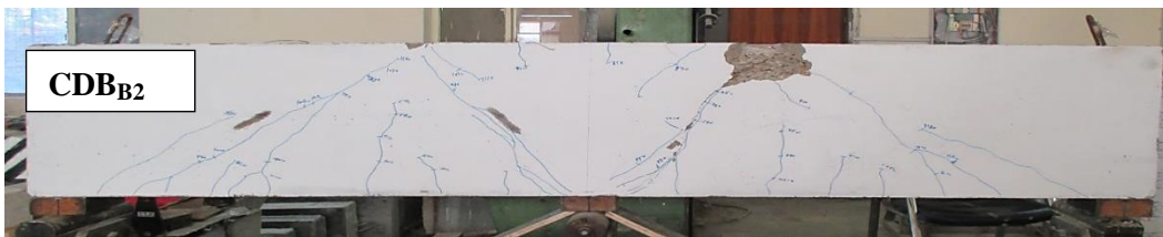
Figure 10. Crack pattern for beam CDB B2 after testing
