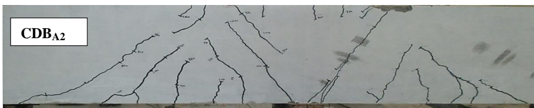
Figure 6. Crack pattern for beam CDB A2 after testing
