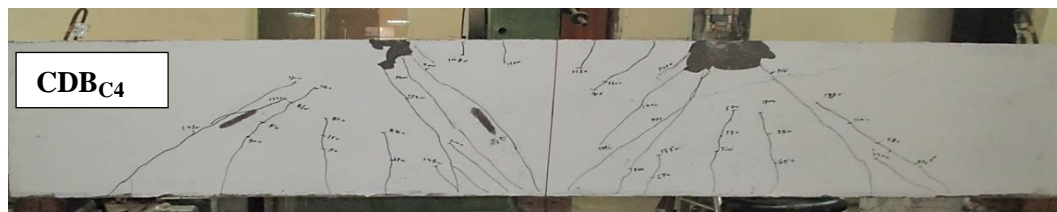
Figure 16. Crack pattern for beam CDB C4 after testing
