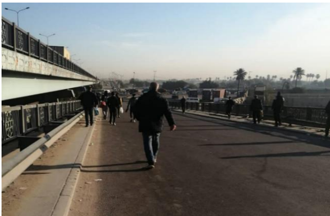
Figure 5. Pedestrian crossing coming from Link C.
