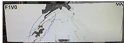
(a) strut crushing failure.
