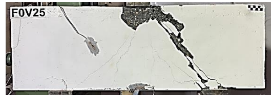
(b) strut crushing failure.
