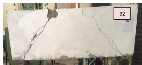
Plate 6. Crack Pattern of Beam 2
