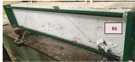
Plate 10. Crack Pattern of Beam 6
