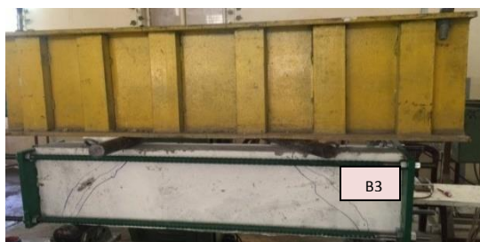
Plate 7. Crack Pattern of Beam 3
