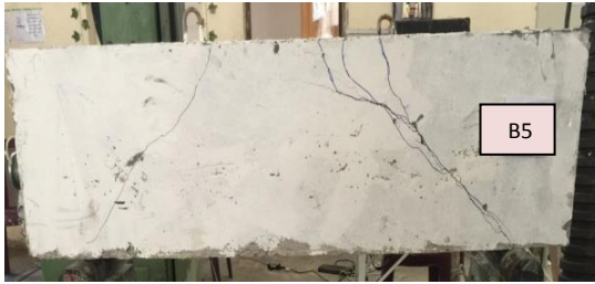
Plate 9. Crack Pattern of Beam 5
