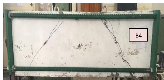
Plate 8. Crack Pattern of Beam 4
