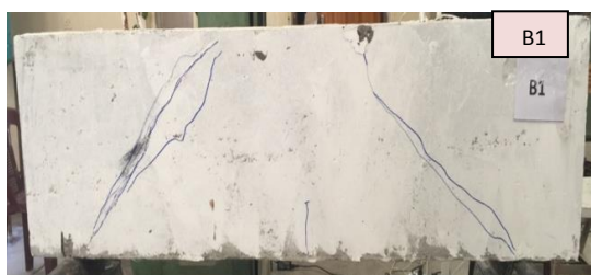
Plate 5. Crack Pattern of Beam 1
