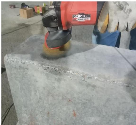
**Figure 2.** Preparing the beam soffit before installing the CFRP sheets
