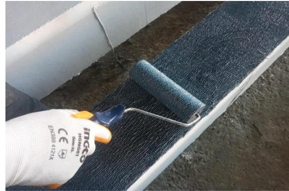
**Figure 3.** Adhering (CFRP) sheets
