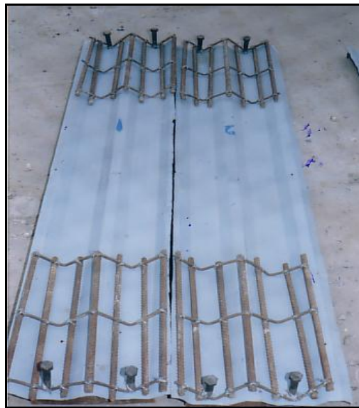
Picture (3) Steel deck with shear reinforcement (RSR)
