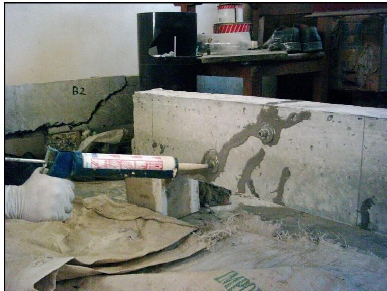
Figure (4) Epoxy injection process
