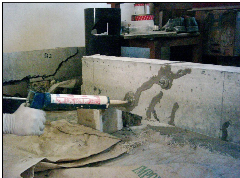
Figure (4) Epoxy injection process
