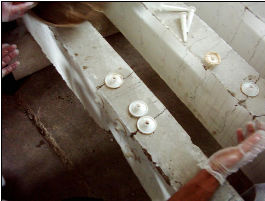
Plate (3) Epoxy injection for beams
