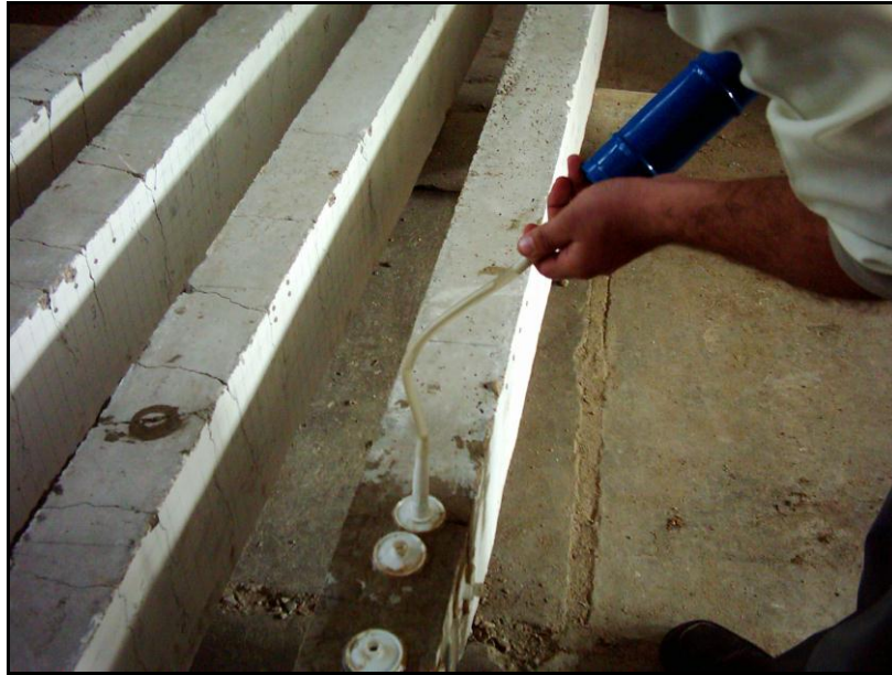
Plate (4) Epoxy injection for beams
