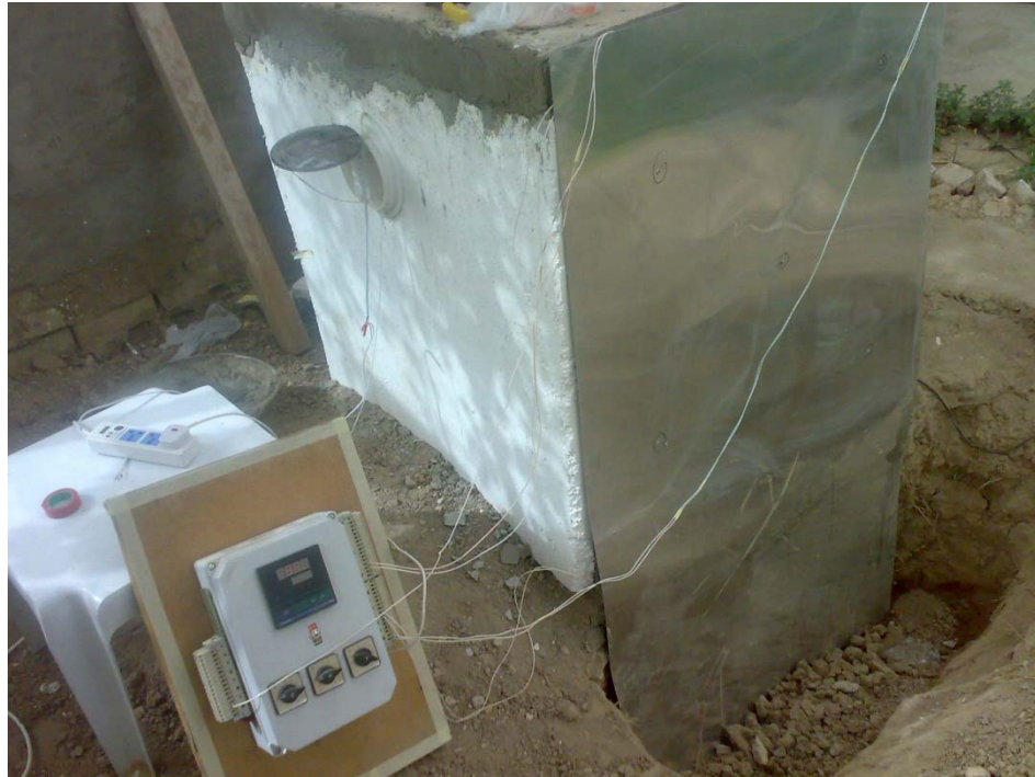
Picture (1): The Metal Sheet Fixed on the Wall.
