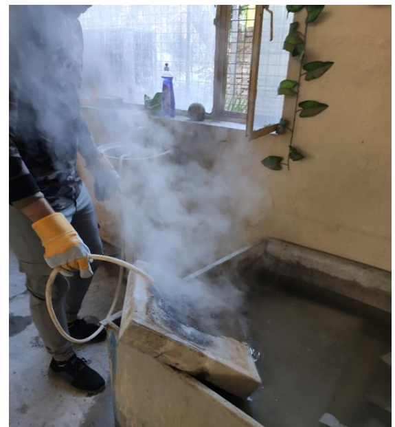
Figure 9. Spraying water on slabs
