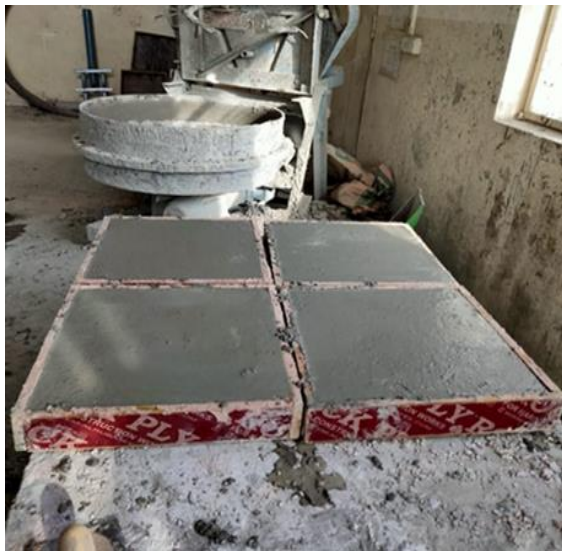
Figure 3. Bubbled reinforced concrete slabs casting
