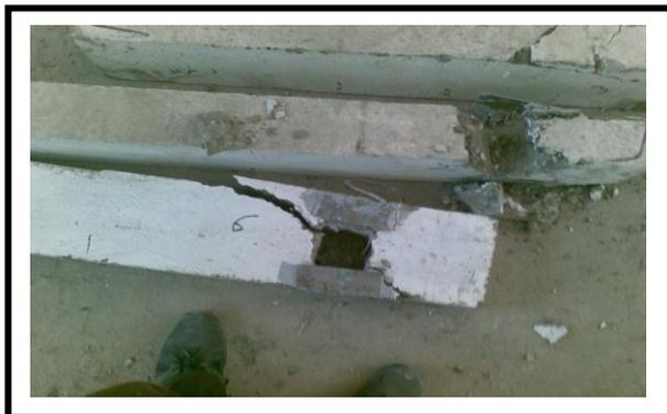
*Crushing of beams*
