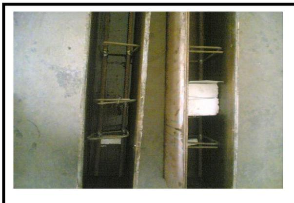
*Reinforcement of beams*
