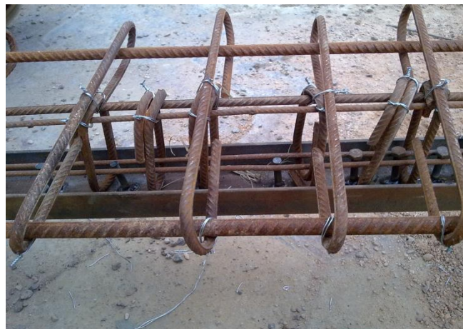
Plate 2: Typical steel reinforcing bar cage resting on the steel channel (with welded headed studs) for a typical test beam.
