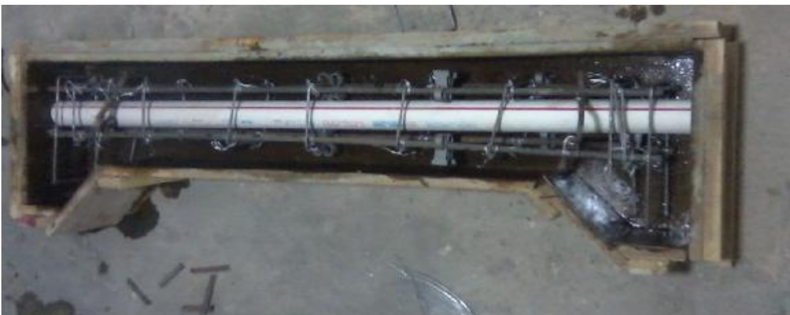
b. Mould of Hollow (PVC Circle) Beam, (B2&B3).
