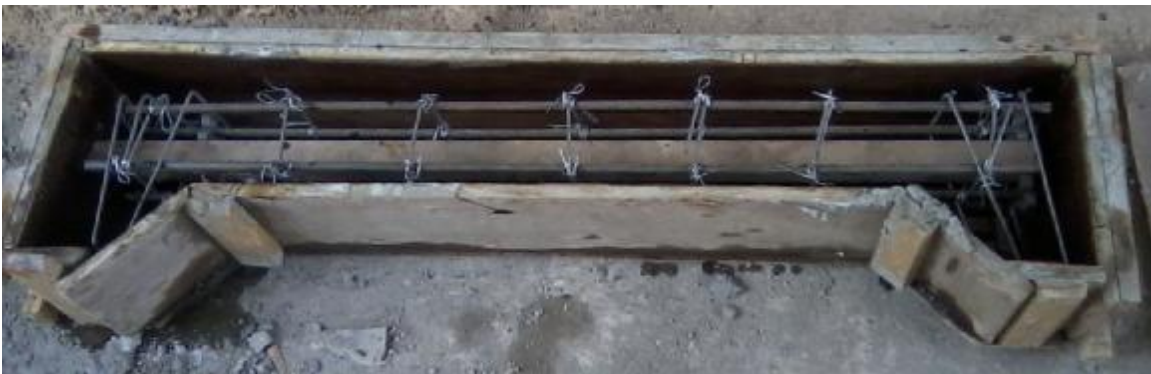
c. Mould of Hollow (Steel square) Beam, (B4 & B5).
